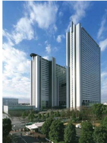
Figure 1.3 NEC Tamagawa plant building
