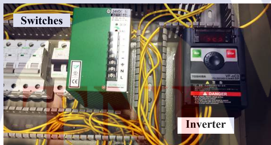
Figure 4.14 The picture of hardware and the inverter model VF-nC3 which control Speed of motor 0.75 kw.
